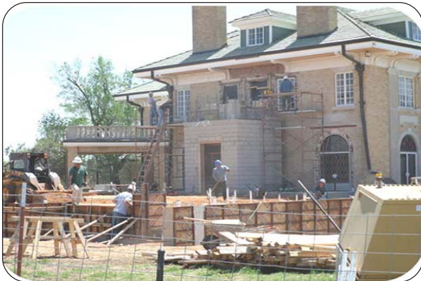
Cushing Valley Hope under construction
