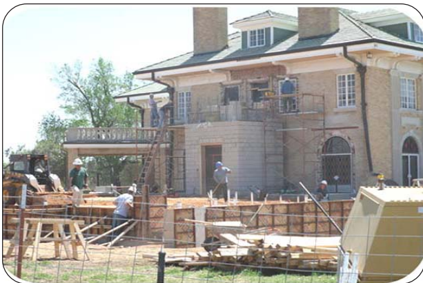
Cushing Valley Hope under construction
