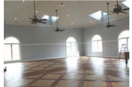
Construction of a great room
